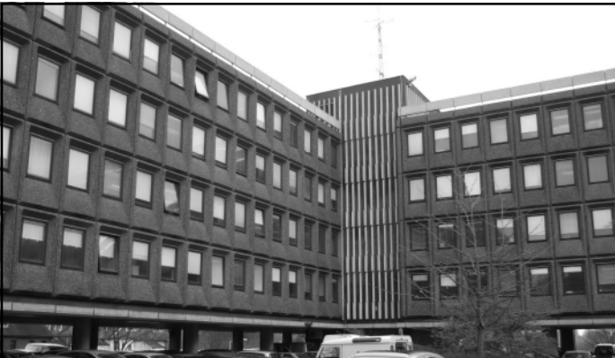
Ashburton Court in Winchester. £40 million was found to refurbish the Tory Council HQ!
