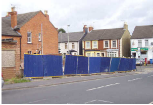
Poor planning control
